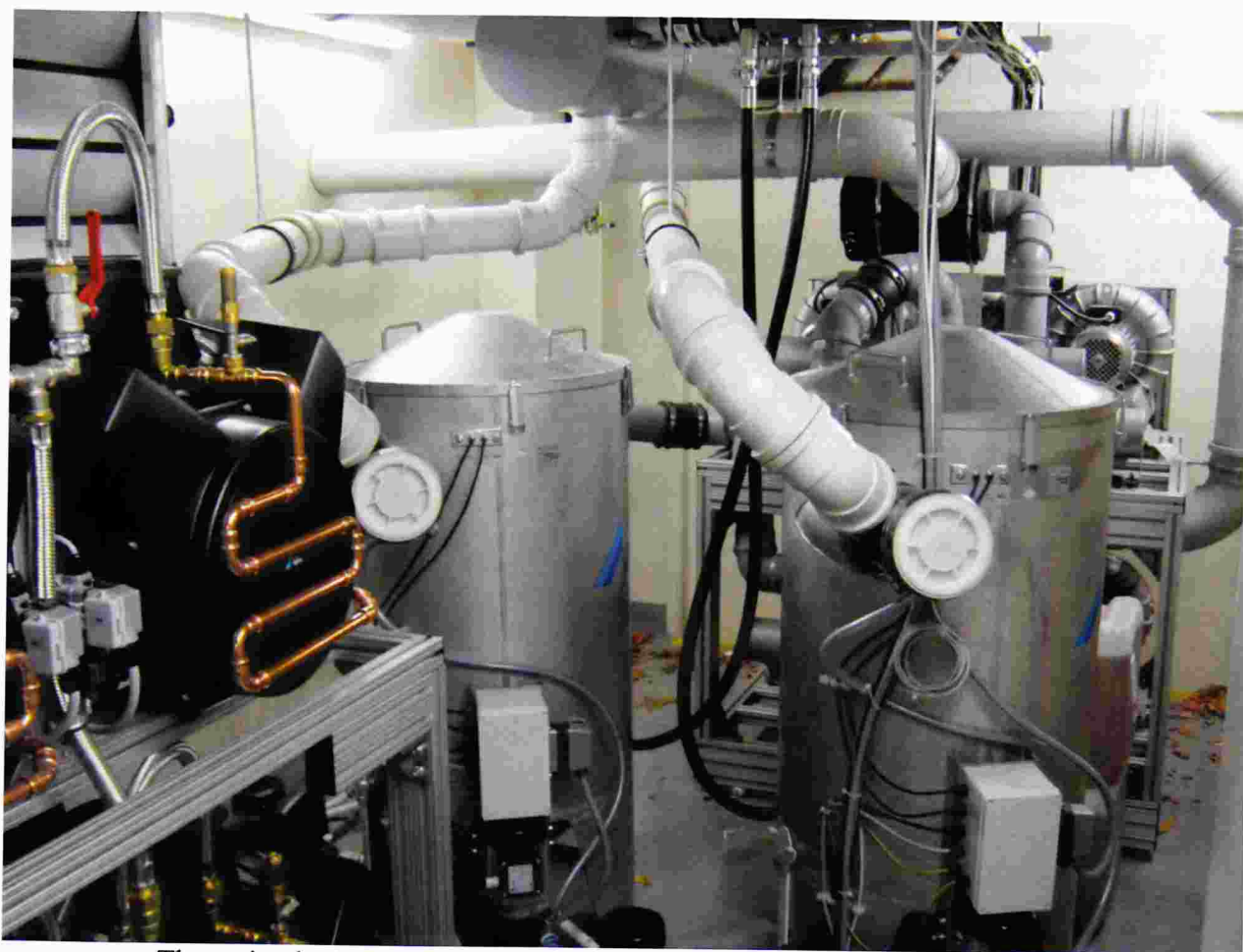
The main plant, compressors to the left, suction separators & vacuum motors
