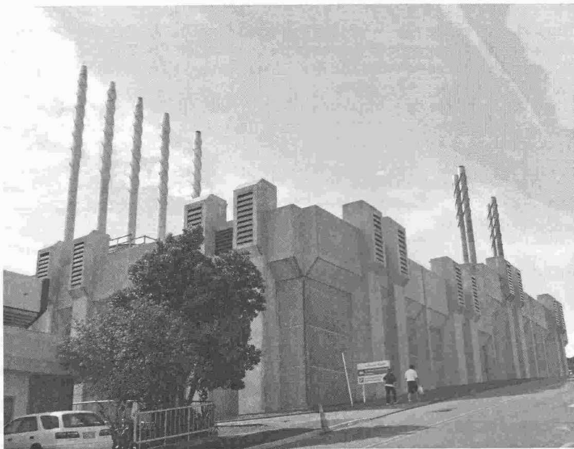
The Wellington Hospital Total Energy Centre rising up out of the steep slope of Mein Street
